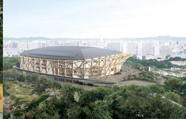
©Aichi International Arena Co.,Ltd.
